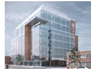
Hostos Community College Allied Health and Sciences Building Complex
