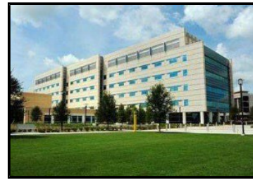
Burnett Biomedical Sciences Building, Health Sciences Campus
